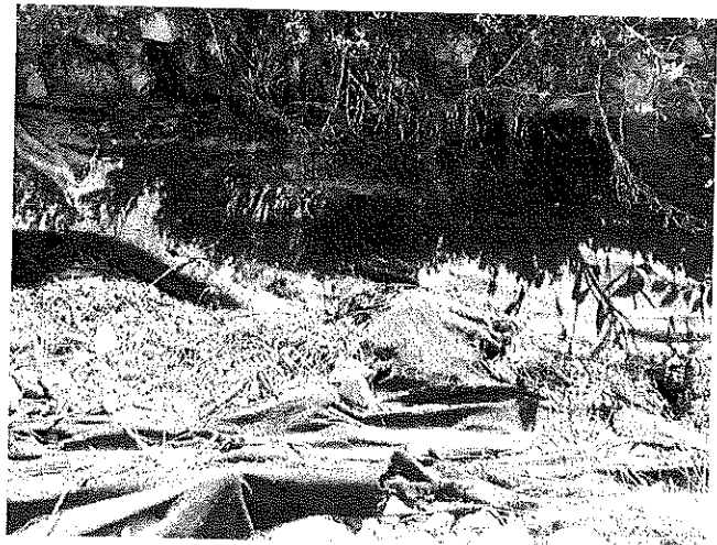
Rock wall has collapsed, exposing the black geo cloth
