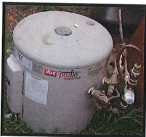
Small hot water cylinder
